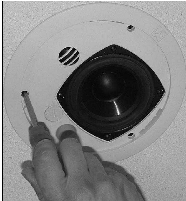
Tightening the swivel-tab screws
